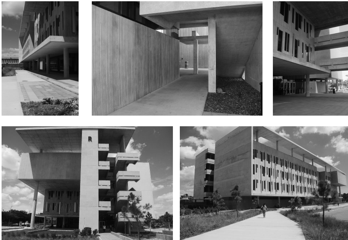
17 through 21 – Building R – 2013 addition to South Campus – Perkins + Will Architects (Photo August 2013)
