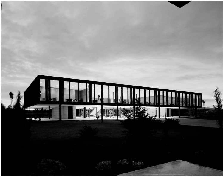
Bacardi y Compañía S.A. Administration Building , Tultitlán, Mexico. Mies van der Rohe with Saenz, Cancio, Martin, Gutierrez (SACMAG) engineers, 1960. Digital print of B & W photograph, c. 1960 Balthazar Korab, photographer. Courtesy of The Library of Congress.
